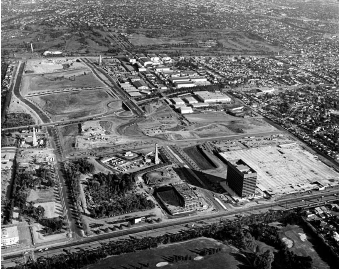
FIGURE 2.11 1963 VIEW OF CENTURY CITY UNDER CONSTRUCTION. This aerial photograph taken in 1963, looking southwest, shows Century City under construction. Gateway West is complete and Gateway East is under construction fronting Santa Monica Boulevard, divided by Avenue of the Stars, which is also under construction. Welton Becket & Associates's headquarters building is in the lower left-hand corner. Source: Los Angeles Public Library Photo Collection
